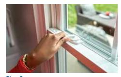
Push the top sash back up to the top of the window frame and the bottom sash to the bottom, then lock the window. Note: If window does not close tight at the center,
