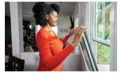
Step 3 While holding the latches in, gently pull the top sash toward you, swinging it down until it rests on the bottom of the sill.
