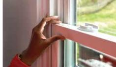
Step 2 Simultaneously slide both tilt latches toward the center of the window.
