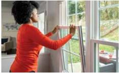
To return sashes to their operating position, swing the sash back up and push the top gently until the tilt latches snap back into place.
