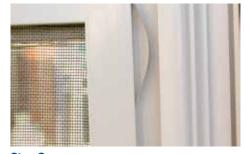
Push the screen to the side containing the screen spring, compressing the spring and allowing the screen to be removed.
